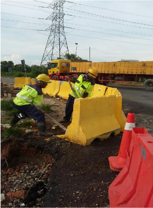
Realigned Concrete Barrier
