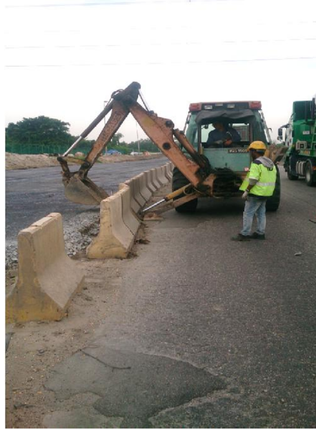
Realigned Concrete Barrier
