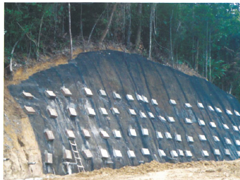
Reinforced Enkamat and Soil Nailing
