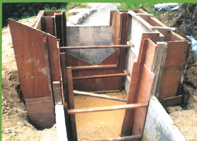
Surface Drainage in Progress
