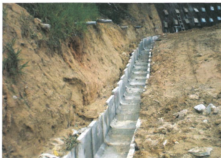
Surface Drainage in Progress
