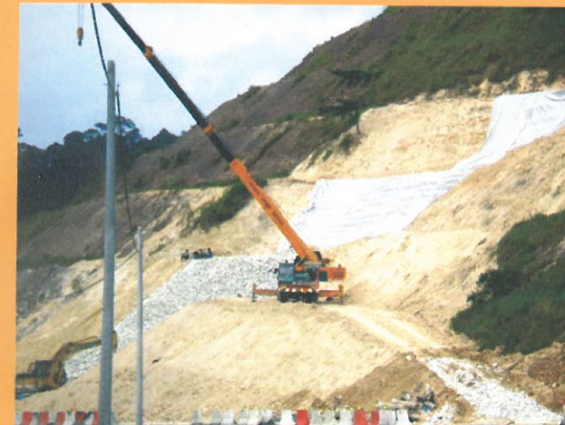
Rock Filling in Progress
