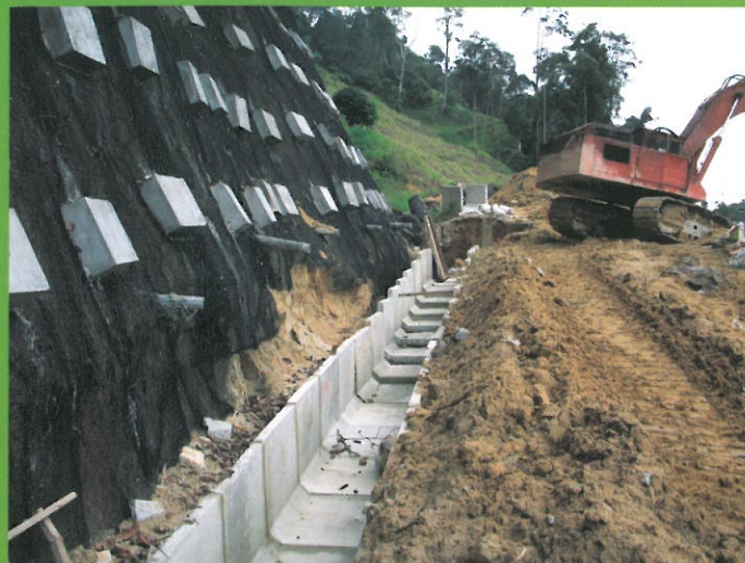
Surface Drainage Works
