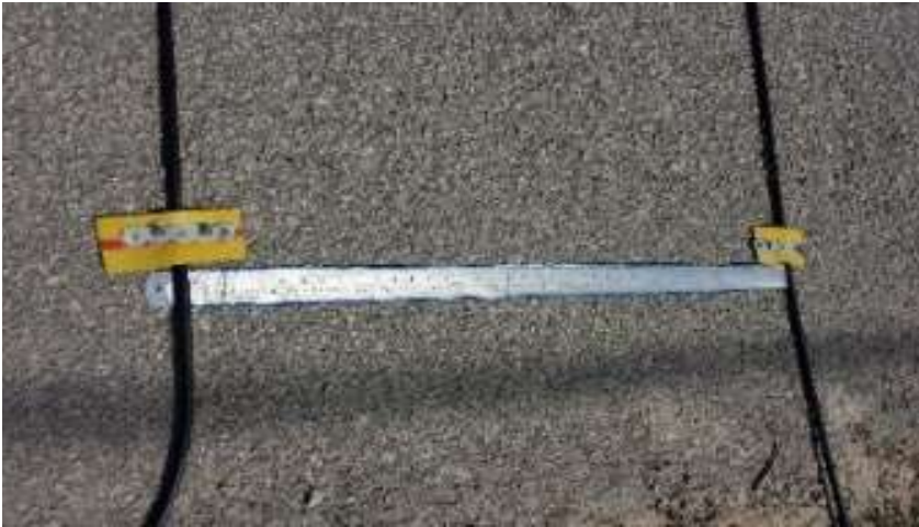
Laying the tubes at 1 meter apart
