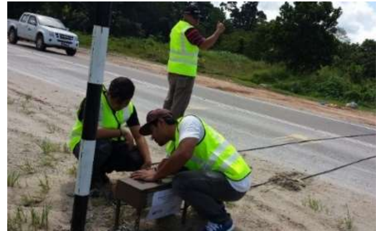
Connecting the tubes to the ATC
