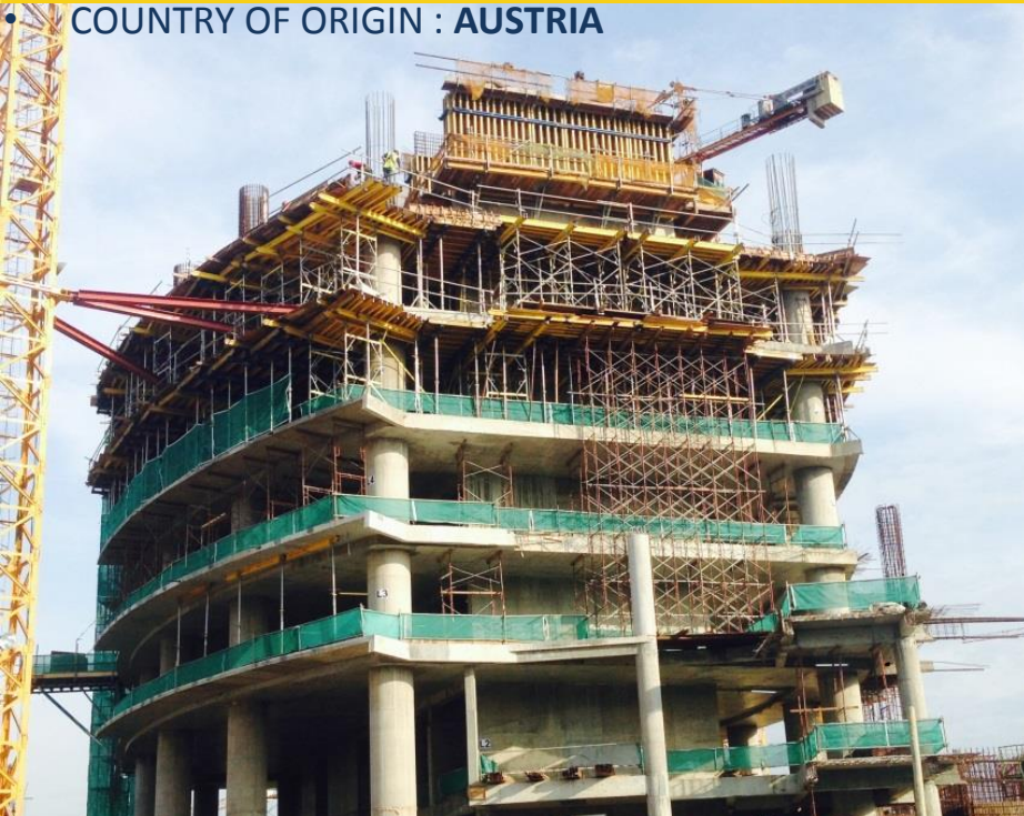
JUMP FORM SYSTEM (CORE WALLS)
