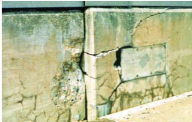
Figure 3: Indicator of ASR sources: (Portland Cement Association Deterioration, Attack, Reactivity, & Defects, n.d.)
