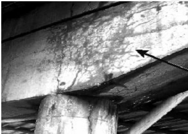
Figure 4: Indicator of DEF, source: CivilDigital.com
