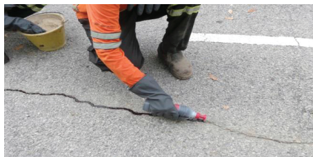
Figure N13: Crack Sealing
