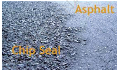
Figure N12: Differential of surface finishing between Chip Seal and Conventional Asphalt
