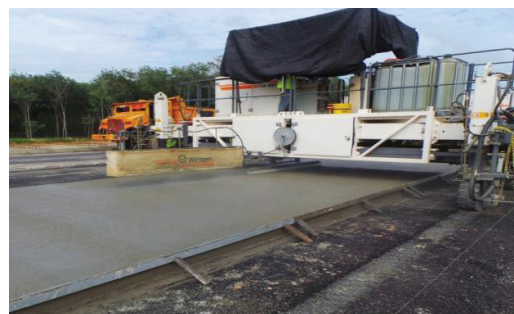
Figure N7: Concrete road pavement under construction
