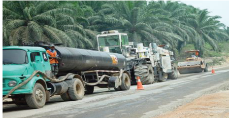
Figure N8: Cold-In-Place Recycling
