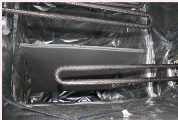
Fig 2. Obstructive Guide Vane Installation
