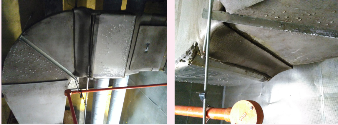
Fig 1. Duct Condensation
