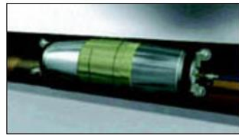
STEP 5: Air pressure is used to deflate the packer. The resin impregnated fibre glass is pressed over the defect and held in place until the resin cures
