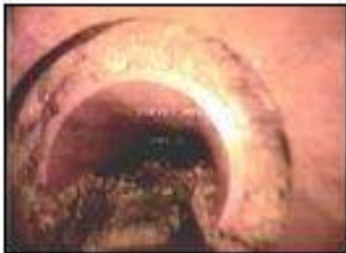
Displaced Joints
