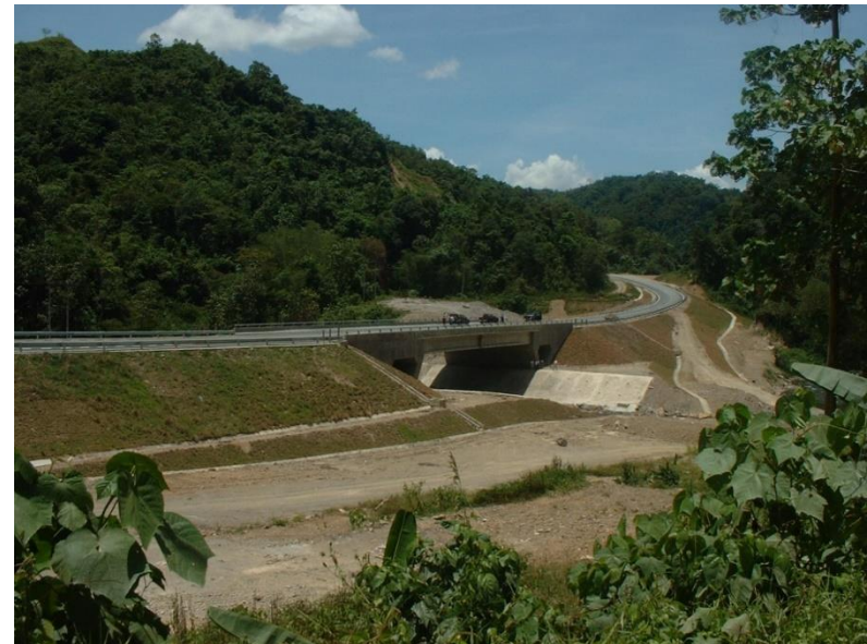
Jambatan Sg Kenipir, Sabah Full continuity at pier - 2004
