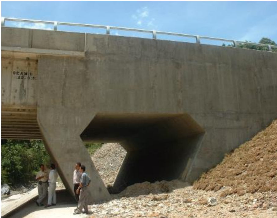
Jambatan Sg Kenipir, Sabah Full continuity at pier - 2004
