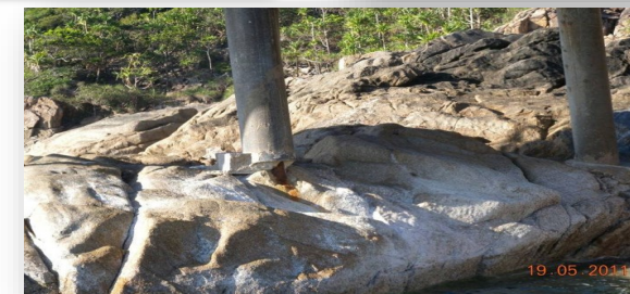
Undermining by flowing water
