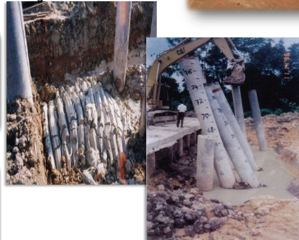
Piling on Soft Ground
