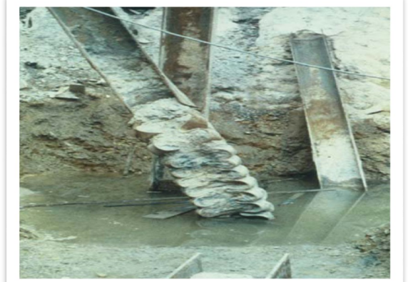
Overdriving of Steel Pile
