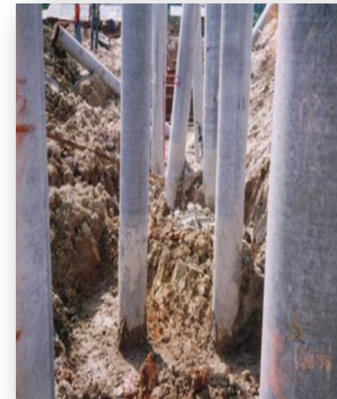
Pile tilted and move away
