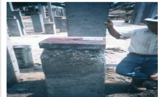
Damage to RC Pile Head
