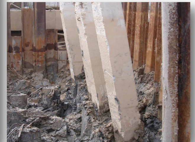
Pile tilted and move away
