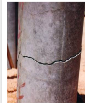
Damage to RC Pile Toe
