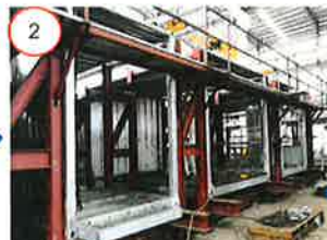
Fabrication and installation off-site
