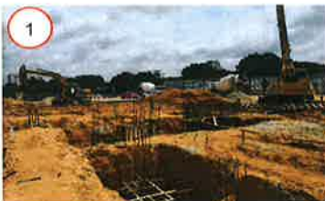
Foundation preparation at site
