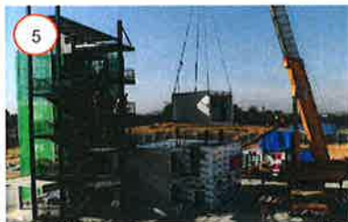
Hoisting, lifting and installation of modules
