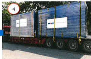
Finished modules delivered to site
