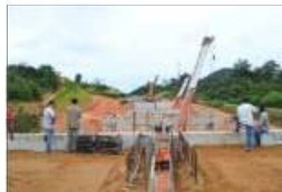
BRIDGE NO 2 – BEAM LAUNCHING IN PROGRESS
