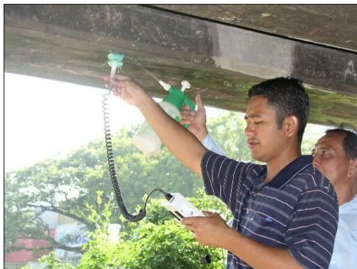
Figure 7.3: Placing the half-cell probe on the concrete surface.
