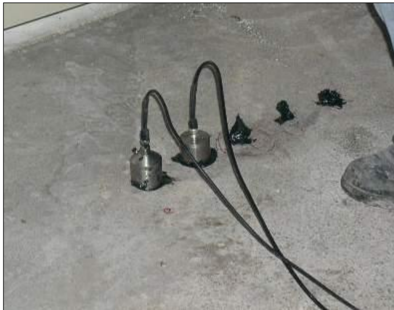
Figure 5.2: Applying coupling agent to transducers and structure surface.
