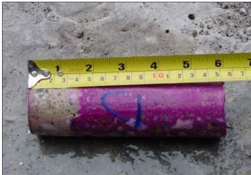
Figure 6.4: Measuring the carbonation depth of a core sample
