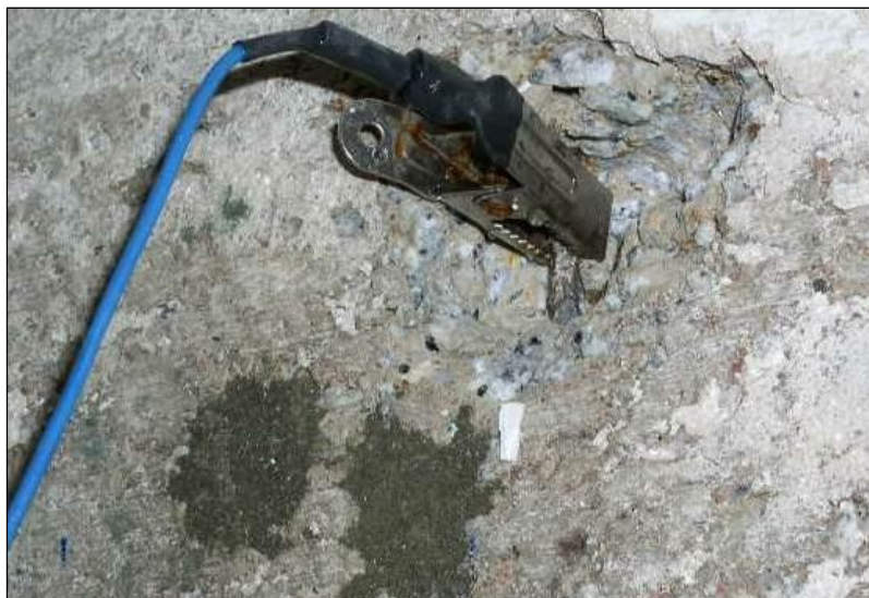
Figure 7.2: Connecting reinforcing steel with crocodile clip.
