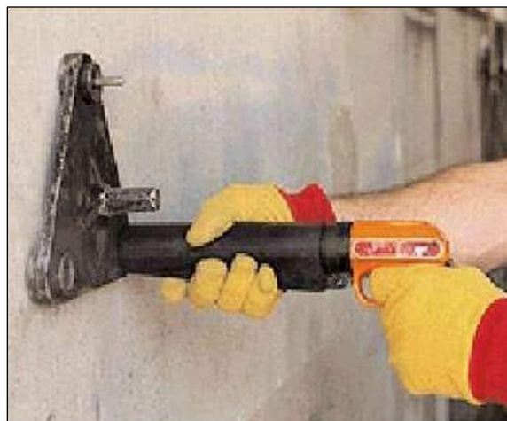
Figure 15.5.2: Positioning the driving unit with probe before fire into the concrete.
