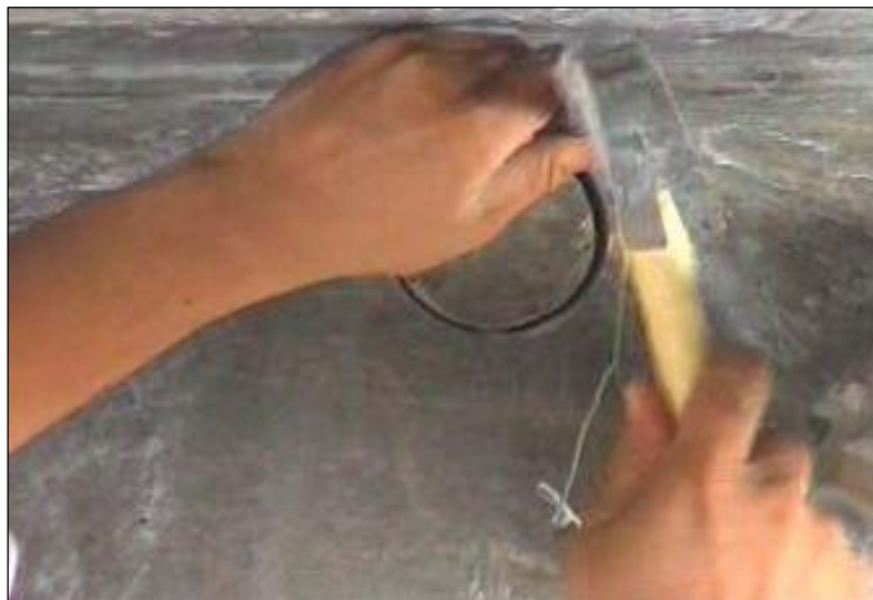
Figure 3.4: Extracting core from the structure.
