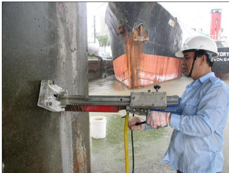
Figure 3.3: Positioning core drill on concrete structure member.
