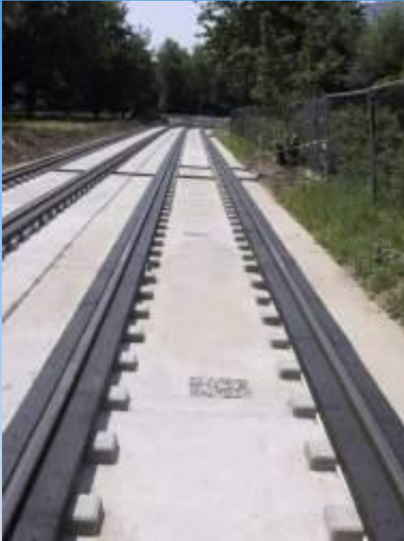
Ballastless Track (Slab Track)
