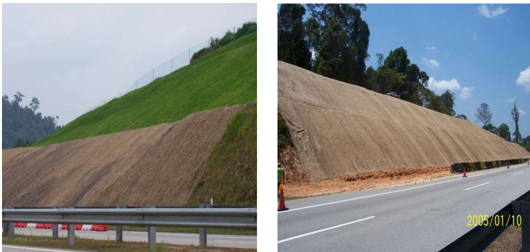
Figure 10: Application of Biodegradable Erosion Control Blanket Layer at Slope
