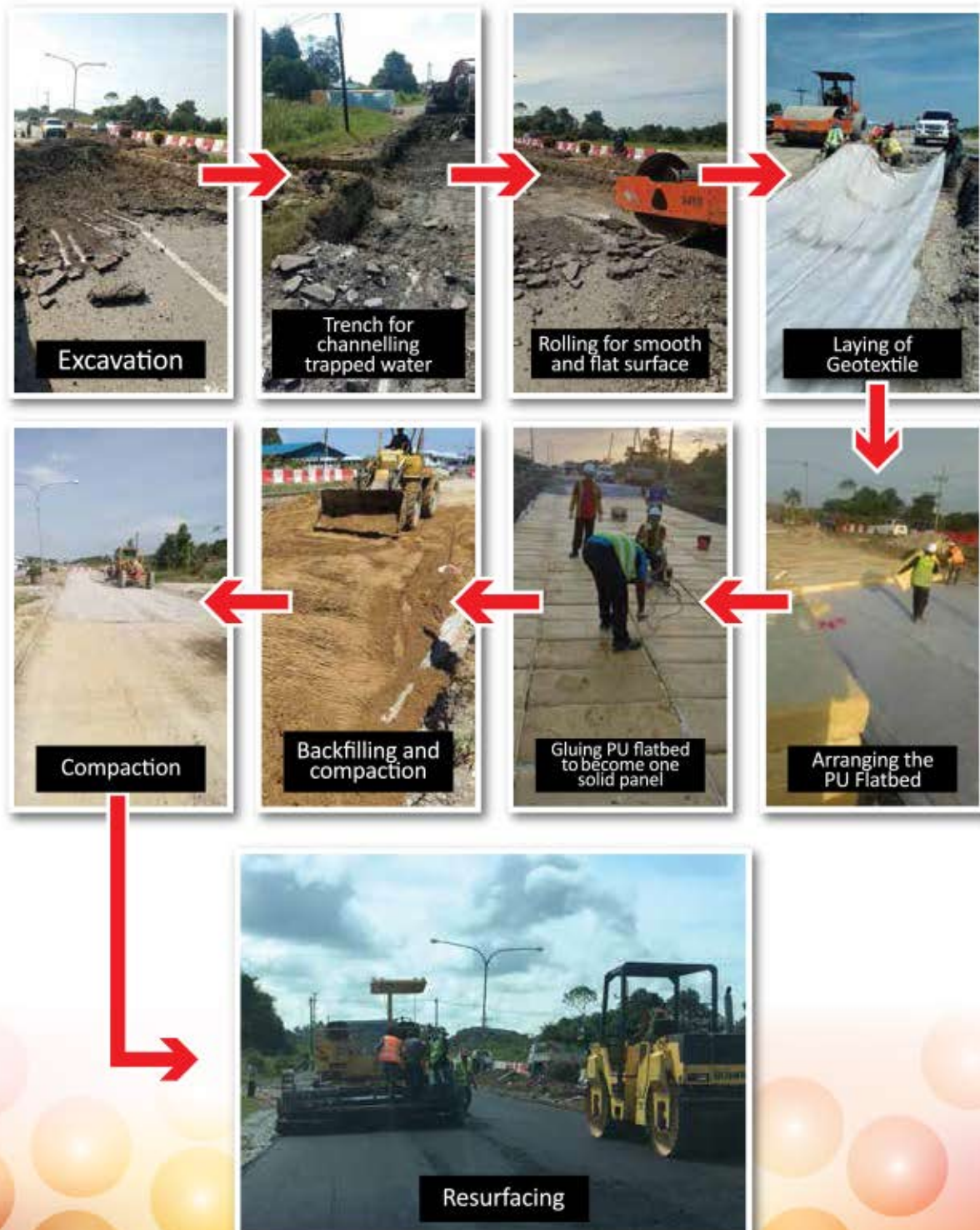
Figure 4. Sequence of construction for the installation of PU flatbed.
