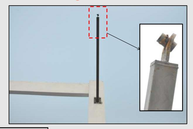
Front strut size was 99.8 mm with 2 mm thickness vs 100 mm with 4mm thickness in construction drawing
