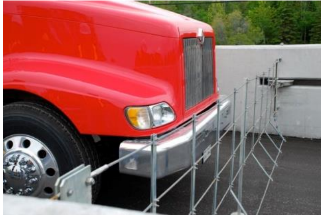
Picture 5.1: A Dragnet system replacing gravel bed arrester (Source: Road Talk - Ontario's Transportation Digest)
