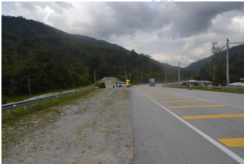
Picture 2.3: Arrestor bed on ascending grade (Cameron Highlands)
