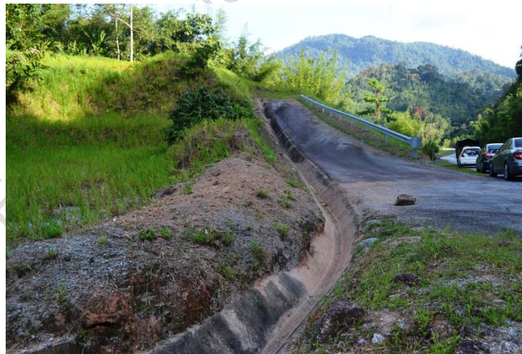
Picture 6.2: Drainage system on ascending grade ramp
