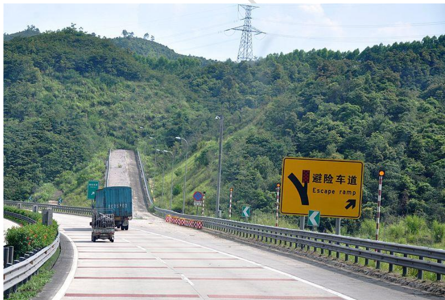
Picture 2.1: Gravity Escape Ramp (Longnan-Heyuan Expressway, China)
