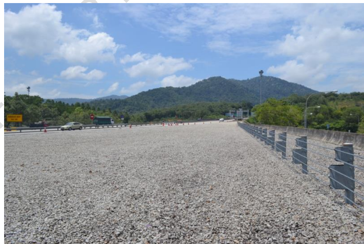
Picture 5.2: A Test Level (TL) 4 safety barrier installed on the sides of an EER (PLUS Jelapang Toll)
