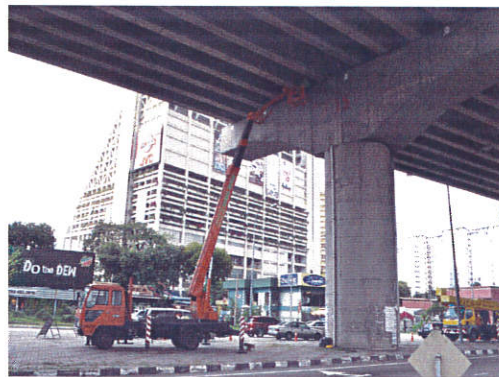
Figure 11: Inspection using skylift
