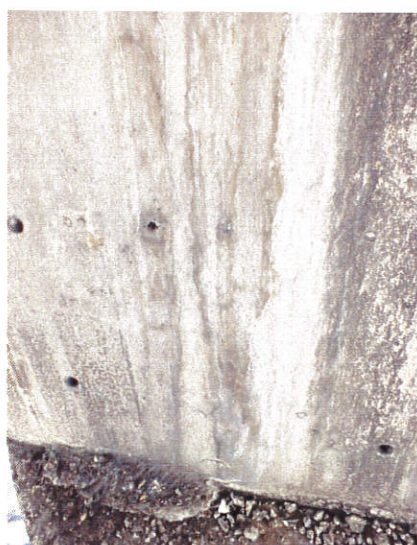
b) Fine vertical crack with width smaller than 0.1mm at the front face of the Pier 14 crossbeam
