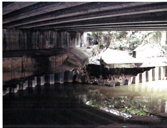
Figure 37: Damaged sheet piles
