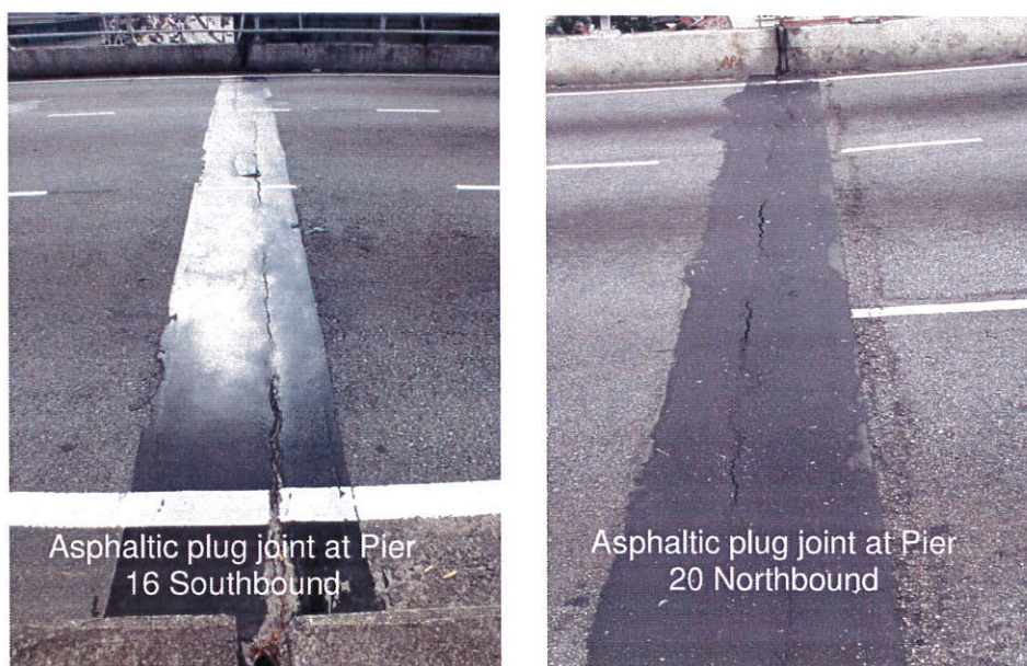
Figure 46: Cracks in asphaltic plug expansion joints
