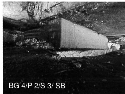
Figure 57: Some bearing that was not in proper contact with the beams
