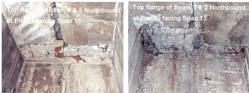
Figure 39: Some top flanges at beam ends that suffered from poor concreting
