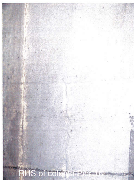
Figure 43: Fine vertical and transverse cracks with maximum width of 0.2mm at right hand side of column Pier 16
