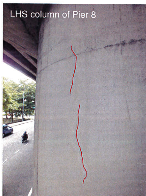
a) Fine vertical cracks at left hand side of Pier 8 column with maximum width of 0.2mm (red line drawn adjacent to crack)
