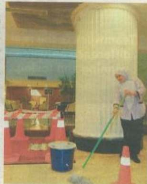
A worker clears a puddle caused by a leak in the roof of Parliament House yesterday. — NST picture by Irfan Adiffin
