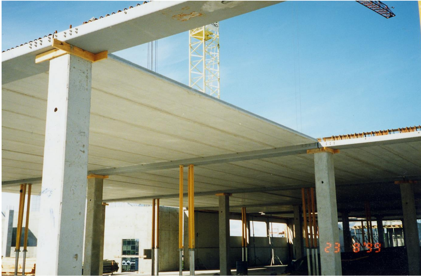
Long span of precast slabs
