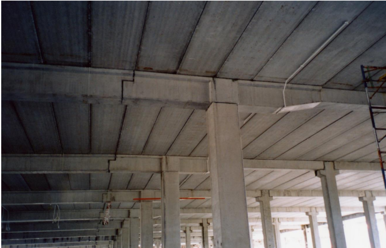
Long span of precast slab
