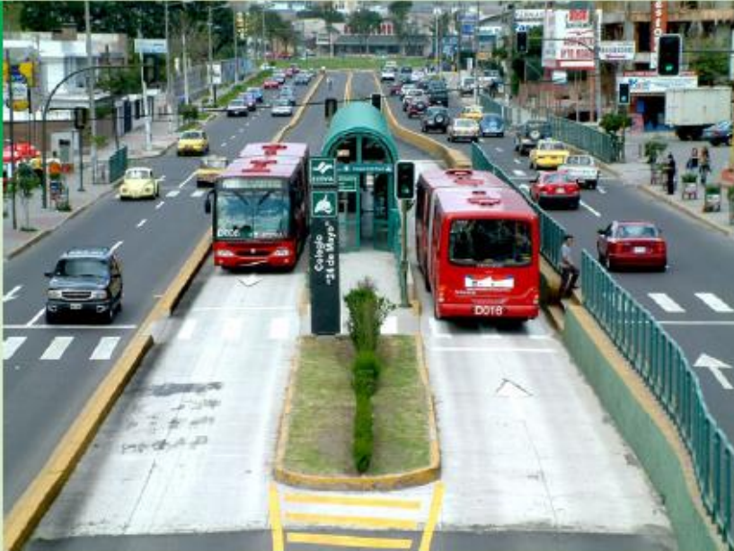
Center stations in the Metrobus Q BRT system in Quito minimize station space requirements and allow easy transfers between different directions of travel.
