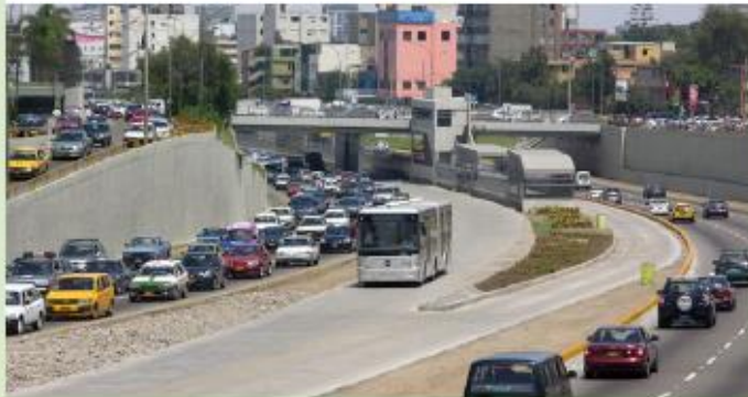
Lima, Peru, uses reinforced concrete over its entire busway.
