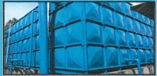
INSTALLATION OF FRP TANK
