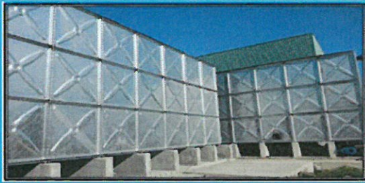
INSTALLATION OF PRESSED STEEL TANK
