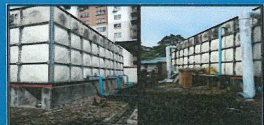
TANK REPAIR AND REFURBISHMENT
