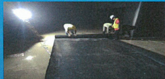
R.C TANK HDPE LINING
