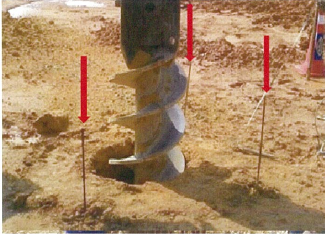
Pancang Besi Setting Out
