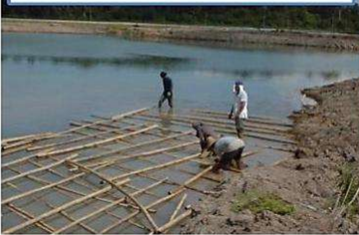
Laying Bamboo Support Structure
