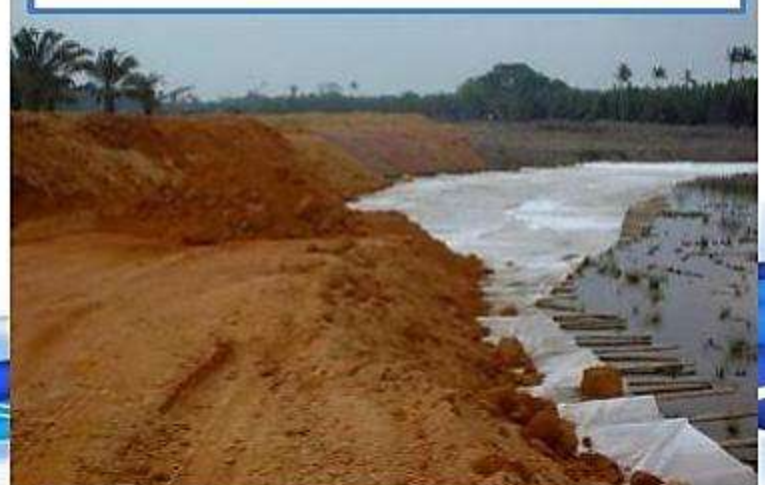
Backfill & Profiling
