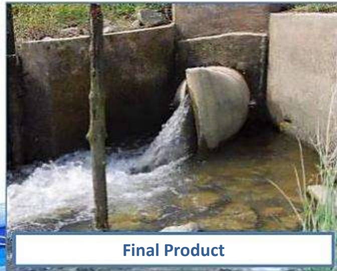
Fitting in Check Valve
