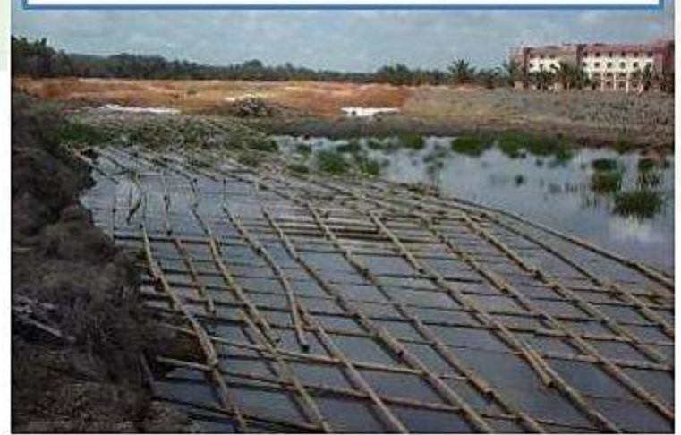
Laying Bamboo Support Structure
