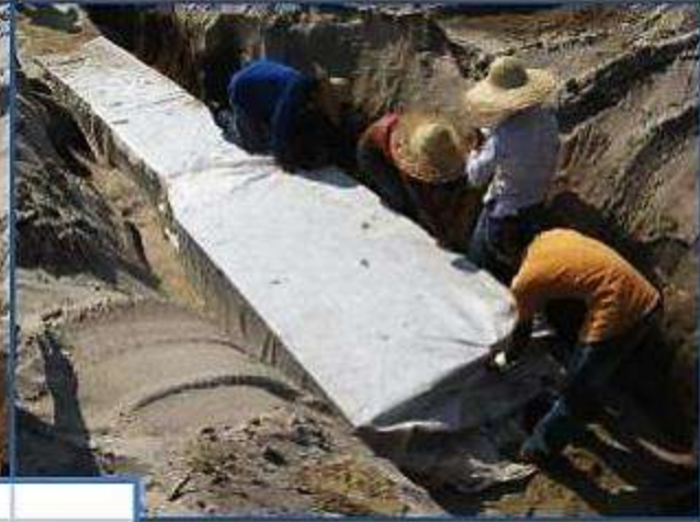
Constructing Subsurface Layer
