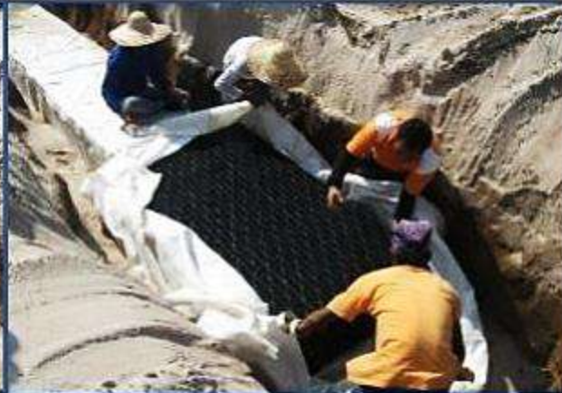
Constructing Subsurface Layer
