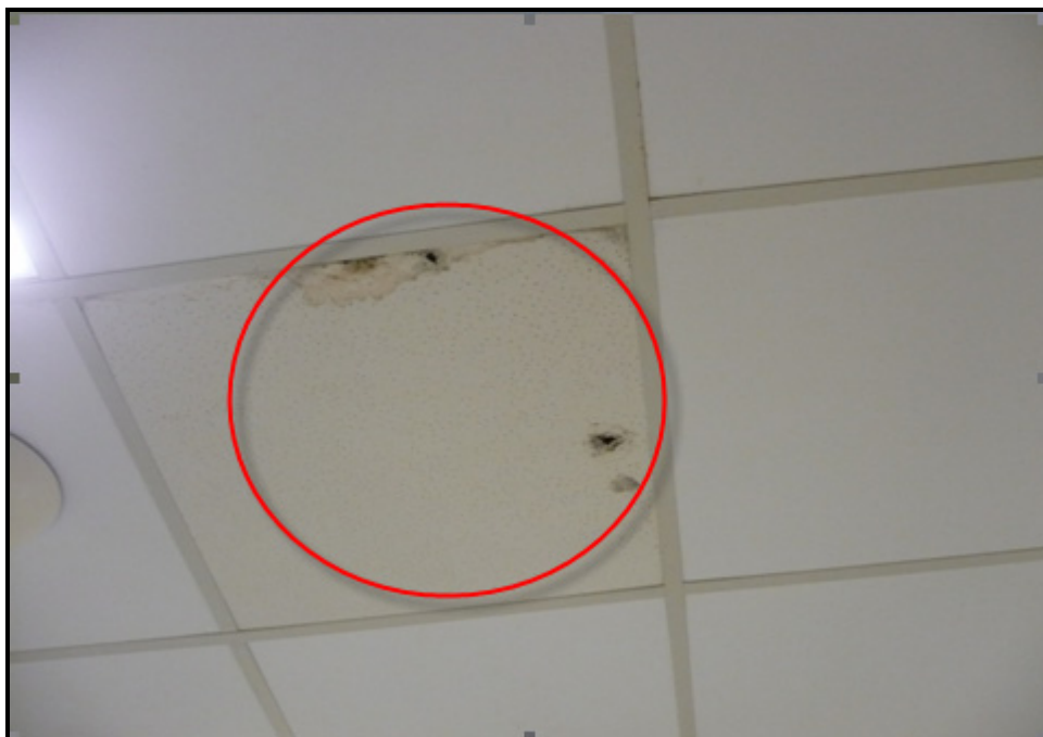
Gambar 6: Keadaan siling berkulat disebabkan kebocoran.
