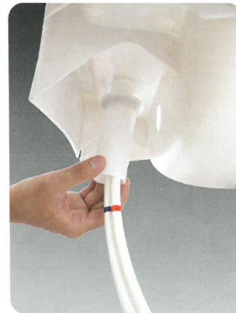
4. Hand-tighten the mixer nut
