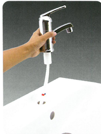
2. Align the basin mixer onto the mounting hole
