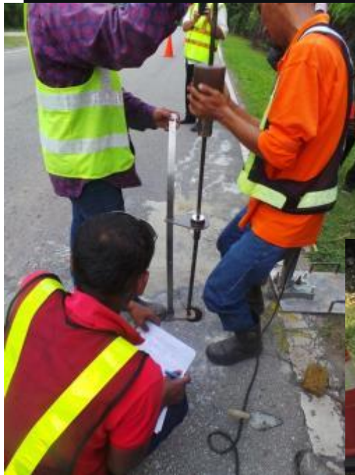
Dynamic Cone Penetrometer
