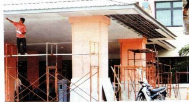
Workers replastering a leaking ceiling at the Sultan Abdul Halim Hospital in Sungai Petani. TOP RIGHT: Workers mapping the floor following a leak which flooded the cafeteria of the High Court complex in Jalan Dutta, Kuala Lumpur, recently.
