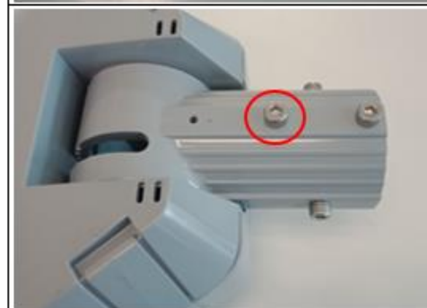
Gambar 4 Road Lighting (LED) - Skru Pengunci Catatan: - L-S 20 Minimum : 2 Bilangan Material : Stainless Steel
