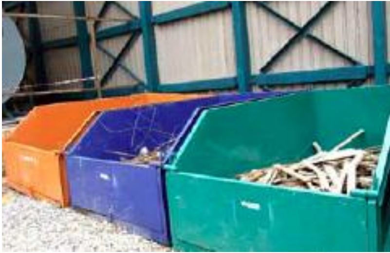
Figure 10: Provide Segregation Bin Construction Waste
