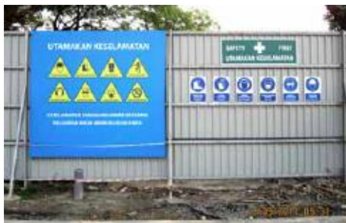
Figure 14: Provide Safety Signage at Scheduled Waste Storage Area and At Entrance of Project Site
