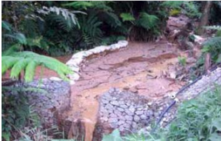
Figure 4: Silt Trap Failure Due To Poor Maintenance and Under-Designed Silt Traps
