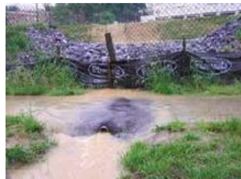
Figure 7: Water Pollution from Sediment Runoff at a Construction Site
