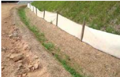
Figure 2: Silt Fence and Earth Drain For Slope Surface Runoff
