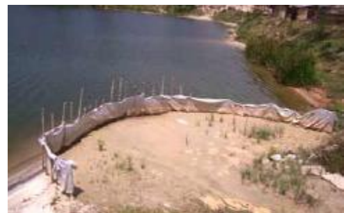
Figure 3: Silt Fence in Sediment Basin for Ease of Maintenance
