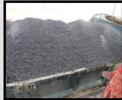
Cuplumps Modified Asphalt
